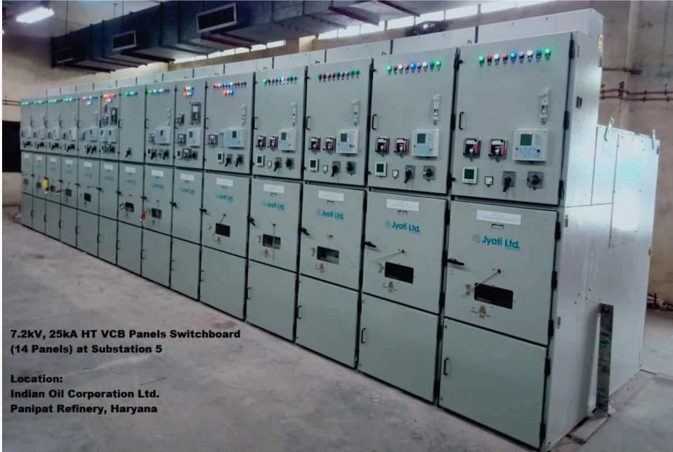
**7.2kV, 25kA HT VCB Panels Switchboard
