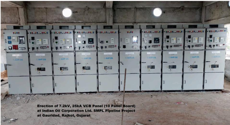
**Erection of 7.2kV, 25kA VCB Panel (10 Panel Board)
